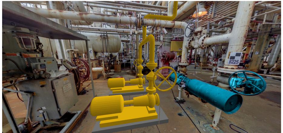
3D scan of a process plant along with imported CAD objects (image is scanned data — not a photograph)
